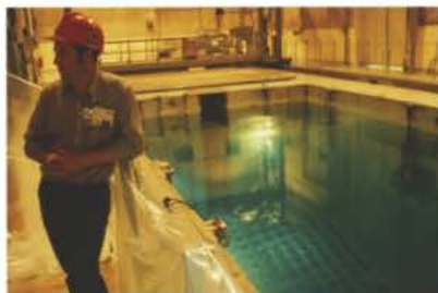
▲ Figure 3 Spent fuel rods in a cooling pond
