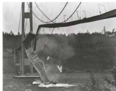
▲ Figure 4 The collapse of the Tacoma Narrows Bridge
